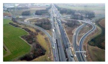
The new flyover bridge has four spans of up to 45 meters and is 172 meters long. The four-lane construction is considered challenging because only a narrow, twometer-wide median strip is available for the supports. But also because the bridge has to withstand enormous and unevenly distributed loads due to its curved course. These are now absorbed by the SMS bearings from SCHREIBER.
