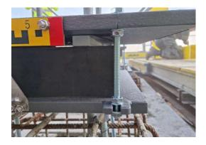
During the construction work, traffic had to be able to continue to flow. Due to the fact that the newly constructed lanes are connected to the existing structure, all bearings were bolted together and can be adjusted in height by means of intermediate plates.
