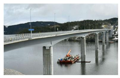
Schreiber Brücken- Dehntechnik manufactured all VS-F 800 expansion joints for the 580 meter long and eleven meter wide steel-concrete composite bridge. These now compensate for expansions or contractions caused by climatic changes and vibrations between the components weighing several tons. They thus ensure the greatest possible safety and stability.
